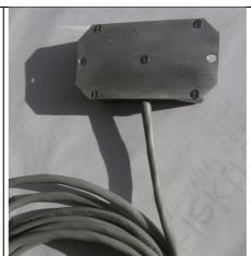
CLF sensor is mounted inside the MV chamber on an earthed panel, and close to the MV cables; mounting should be above or next to one of the outer phases.
